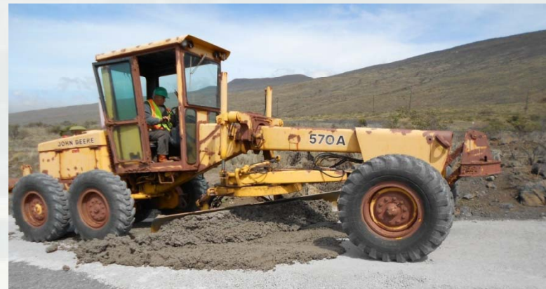
Spreading for roller-compaction
