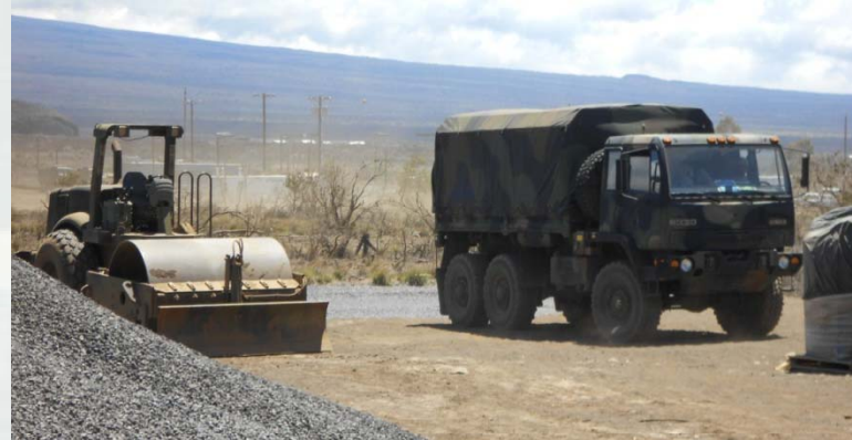
On-site equip. for placement
